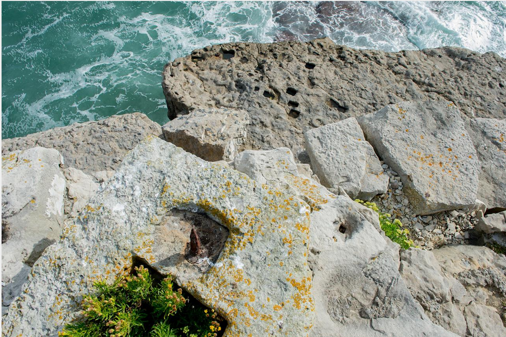
Rusted gudgeon pin belonging to the gibbet used to lower the stone to the lower loading rock. On a slab of Blue Bit thought for strengthening.
